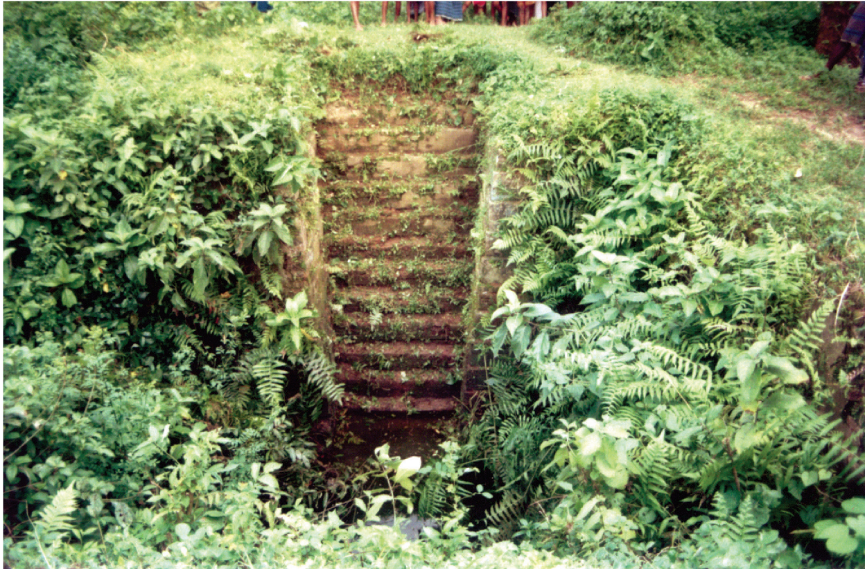
Figure 6: Close-up of the descending steps of the well (Baoli) of Yogir Bhavan
