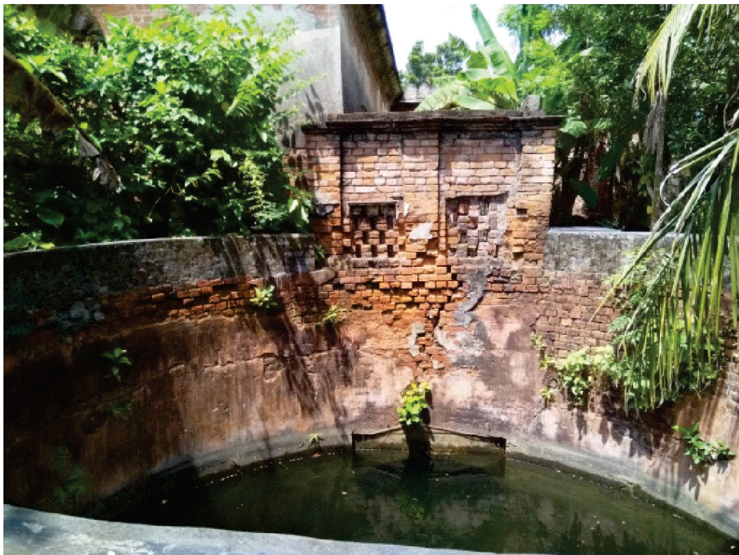
Figure 14: View from opposite side of the staircase
